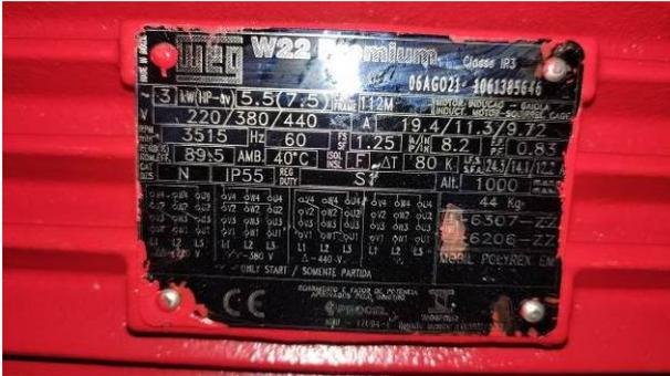
Figura 19E: Bomba hidrantes (plaqueta motor)
