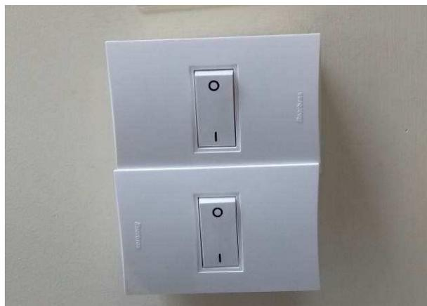
Figura 18: Interruptor bipolar simples
