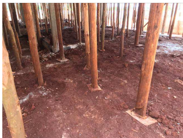
Figura 01C: Reaterro entre as vigas baldrames.
