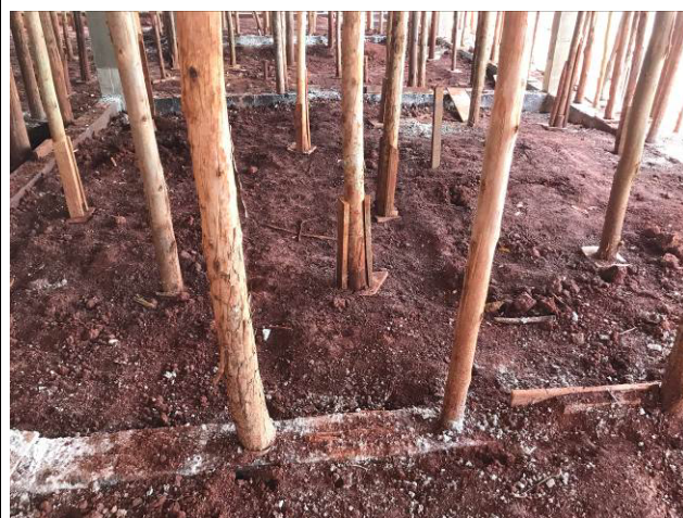
Figura 02C: Reaterro entre as vigas baldrames.
